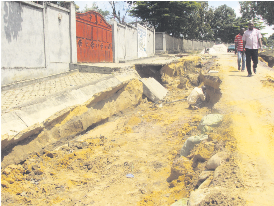
La route de la station terrienne
