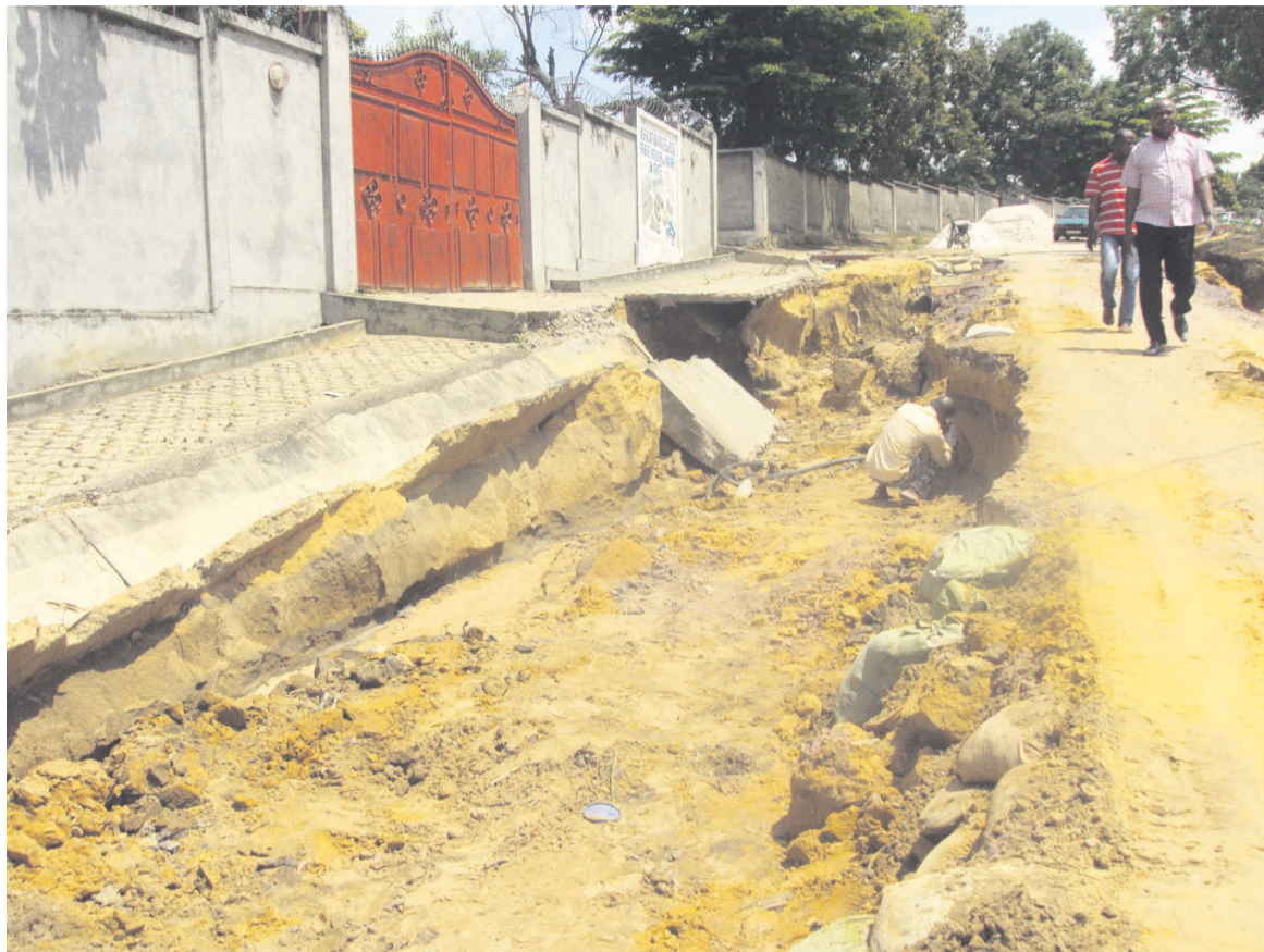
La route de la station terrienne
