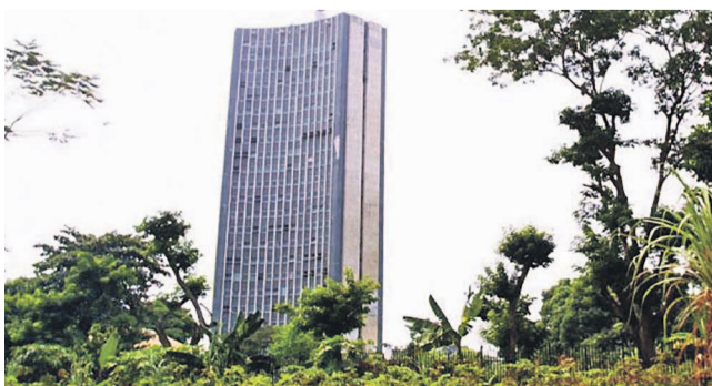
La tour administrative de la RTNC
