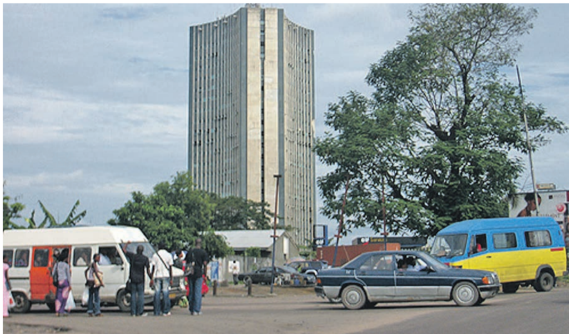
La tour administrative de la RTNC
